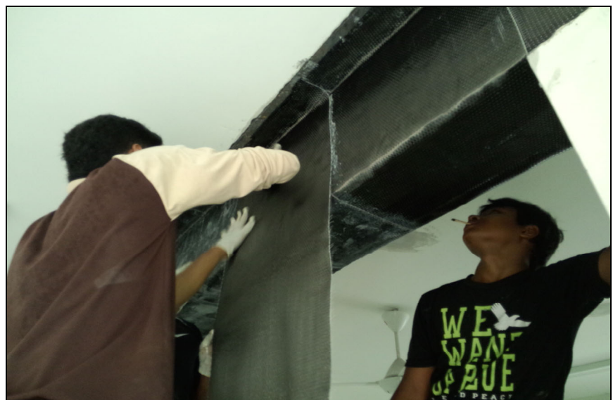
Apply of Build Wrap AAA 300 on Beam
