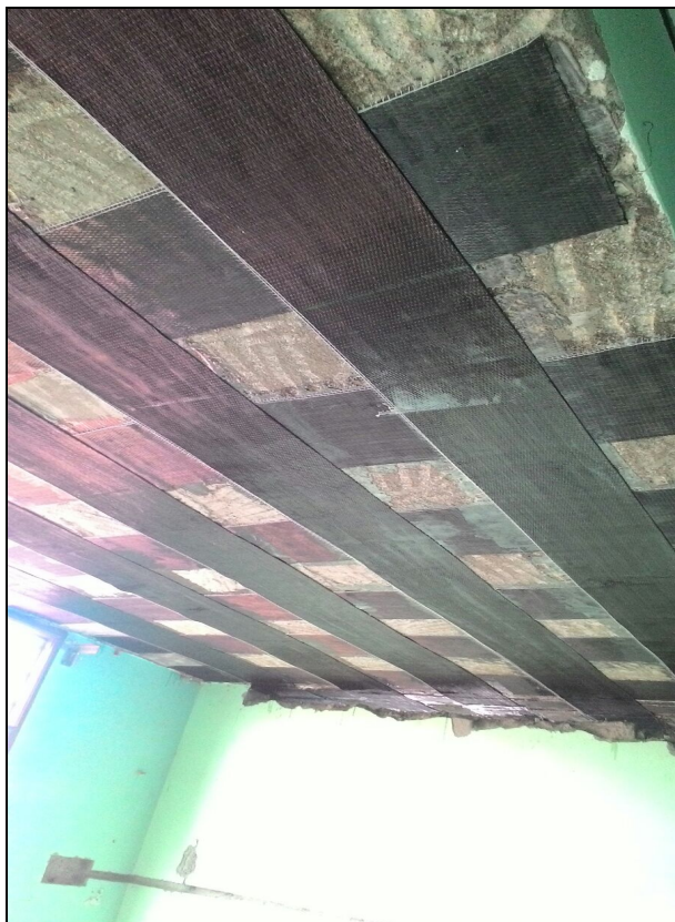
Build Wrap AAA 300, apply on Slab
