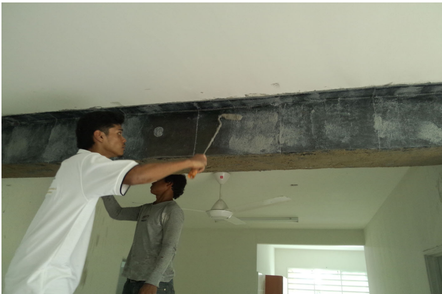
Surfaces Preparation, Apply of Epoxy Primer
