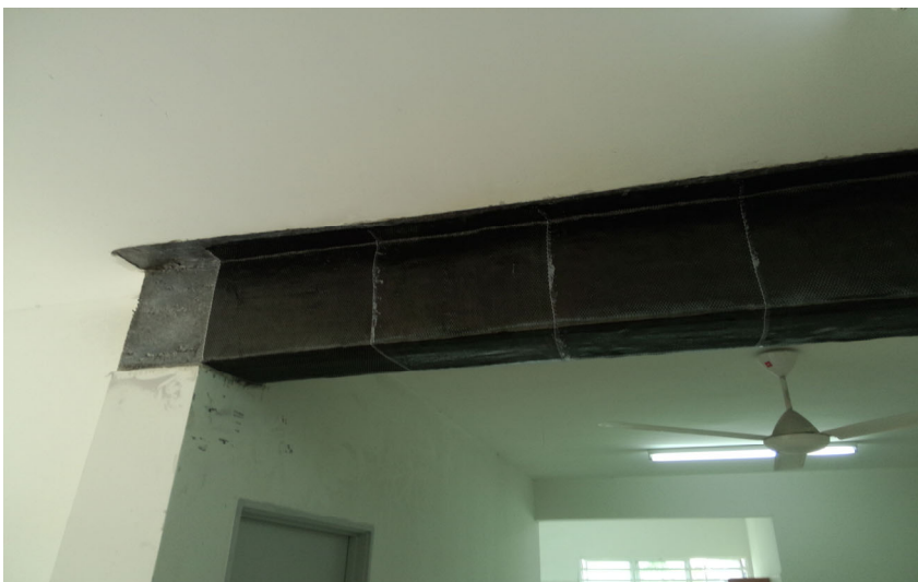
Completed Apply of Build Wrap AAA 300
