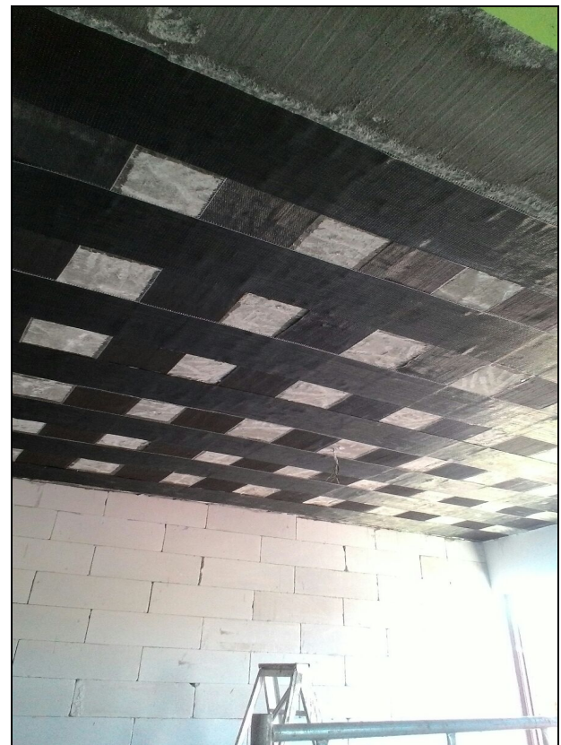
Build Wrap AAA 300, apply on Slab
